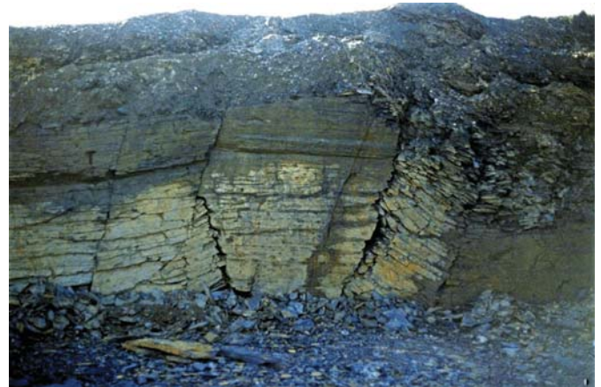
Fig. 3. Abandoned, partially collapsed deep (under-ground) bituminous mine; Clearfield County, PA; 12-22-88. Typical room and pillar pattern is shown. The undisturbed block is where the coal pillar is intact. On either side of the pillar, the rooms have collapsed. This collapse is called deep-mine subsidence. When this deep mining occurred, equipment did not exist that made it economical to strip (surface) mine down to the coal. Abandoned deep mines can be problematical. Commonly, the subsidence can work its way to the surface, even when the coal is 800 feet below the surface as with the Pittsburgh coal. When the subsidence nears the surface, it can affect structures such as houses and roads. Half of Colorado Springs, CO. is underlain with abandoned deep coal mines.
