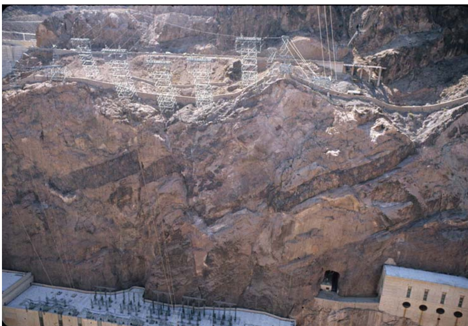
Figure 2: En echelon normal faults in the abutment at Hoover Dam.
