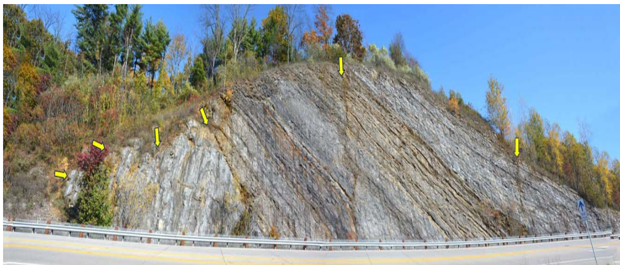
Figure 2: Panorama composite of the Scotia/Grays Woods I-99 interchange roadcut. The faults are inferred splays of the Birmingham Thrust Fault. Image by the author.
